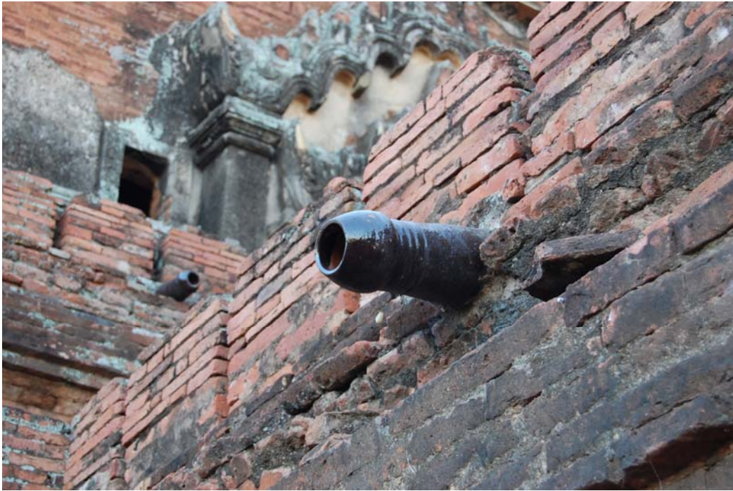
Additional drainages from the roof terrace
