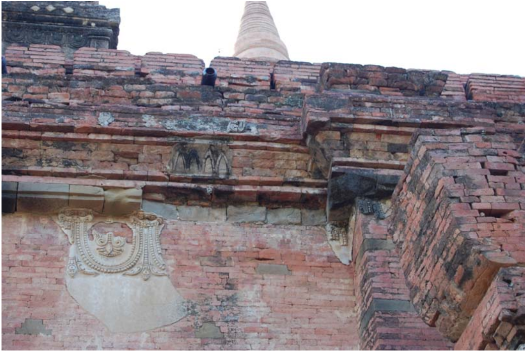
Lack of members from the cornice level of a wall
