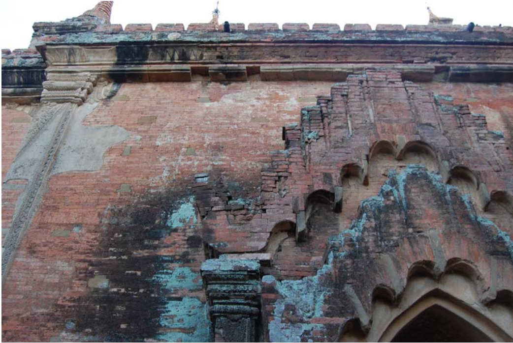
Growth of microorganisms on the wall
