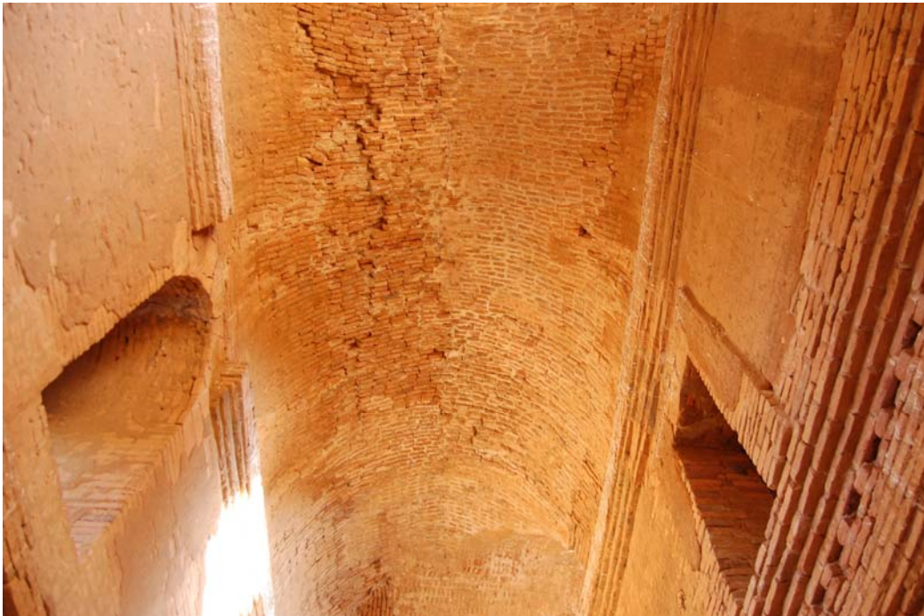
Horizontal crack on top of a vault
