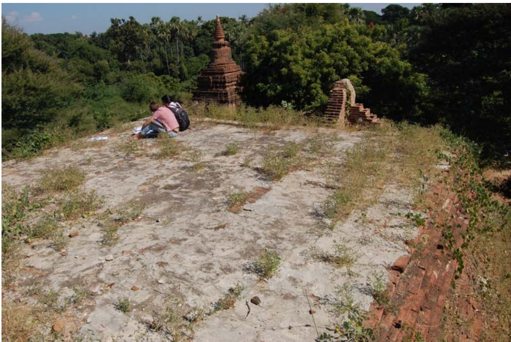
Deteriorated surface of the roof
