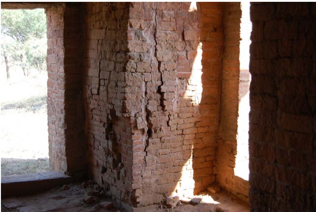
Breakage around a wall corner
