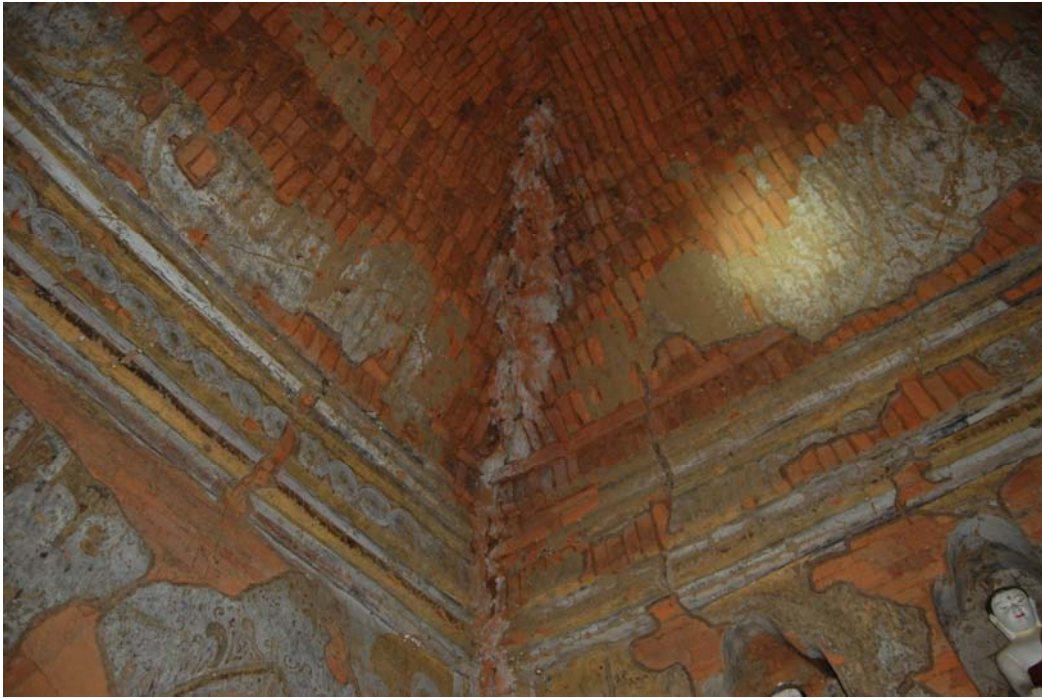
Trace of water leakage at the corner of vaulted ceilings
