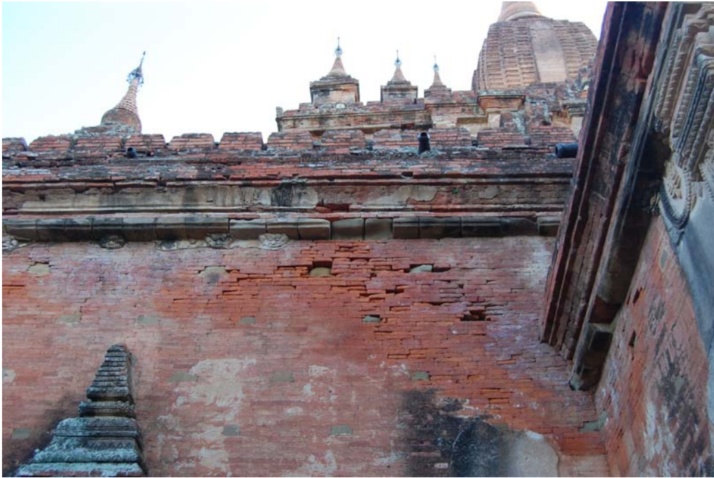
Deteriorated surface of a brick wall
