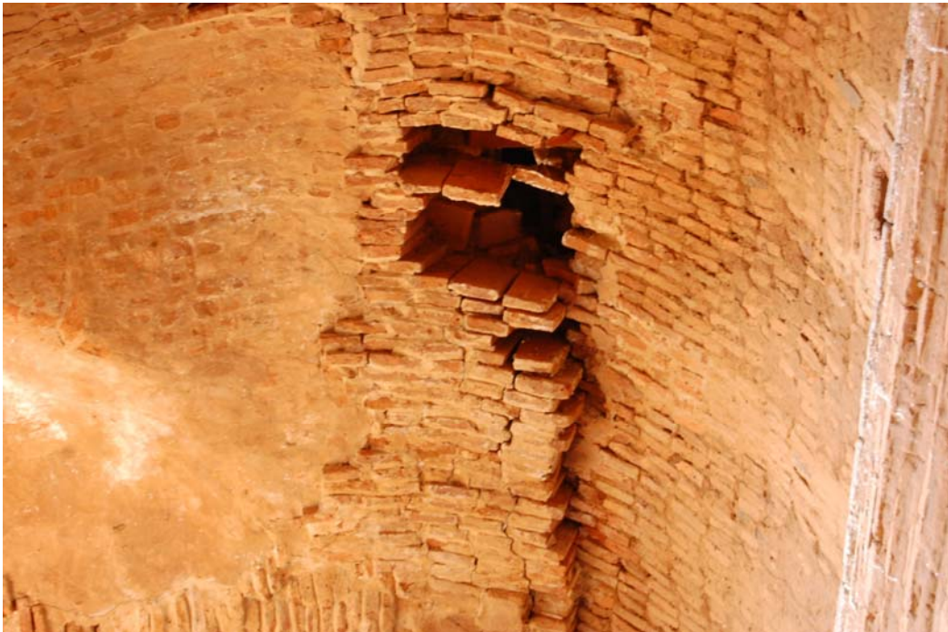
Lack of bricks from a vaulted ceiling
